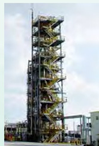
Figure 5: HS-FCC Demonstration unit
