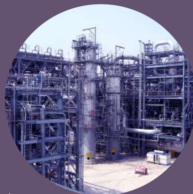
↑ SRU with Sultimate™ Tail Gas Treatment Unit (TGTU) 2x300 TS/d, 99,9 % sulfur recovery India
